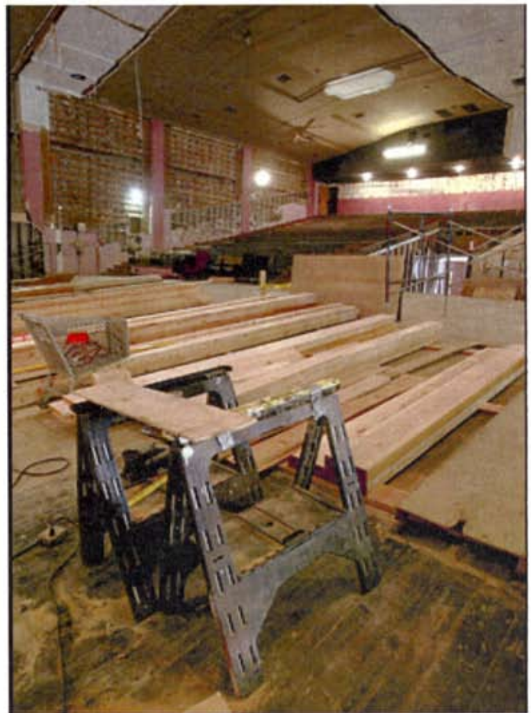
Renovations are under way on the interior
